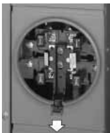
Manual Slider-Type Bypass Shown in Closed Position with Handle Extending through Notch in Rim of Meter Socket Cover
