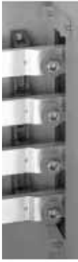
Captive Equipment Bonding Screws are Located on Right Side of Each EZM Main and Branch Device
