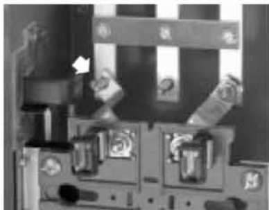
Step 1: Remove hex nut from A \phi line side connection to vertical bus.
