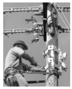
Secure cluster mount to pole using double-arming bolts.
