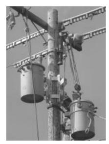
Transformers may now be installed using enclosed bolts, washers, and nuts as shown in Figure 3. Install ground wire between the two stainless steel wire clamps provided on one of the bodies.
