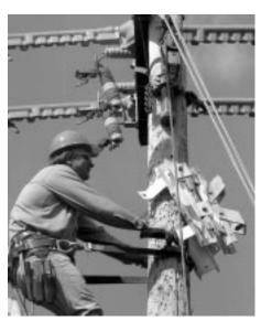
A Note which of cluster mount body extrusions has a mounting key hole and install 1/2" lag screw in corresponding position in pole. Hang cluster mount on lag screw.
