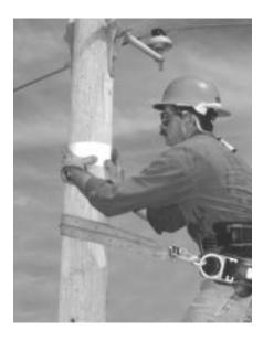
Measure pole at mounting height with enclosed pole measuring tape. Tape will show proper notch for hook plate adjustment.
