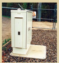
QUAZITE® cell site enclosures allow cellular providers easy access to their cable lines and provide plenty of room for the addition of new lines. Sixteen 4" terminators enable providers to easily add new feeder cables to existing sites. The terminators also reduce the risk of disturbing existing service when adding new cables because installers can clearly see where other cables are entering the box.
