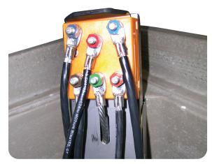
Bonding Harness Or Locate Wires
